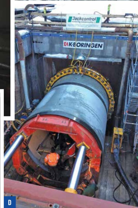
and, with a tight radius of 259 m, the MTBM was brought approximately 1.0 m closer to the surface than initially planned.
