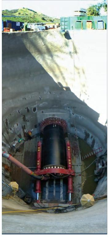
PRIOR TO CONSTRUCTION, THE CONSTRUCTION TEAM PROPOSED Combining multiple drives into a single, long s-curve drive that would eliminate one shaft and convert another to a push-through shaft.
