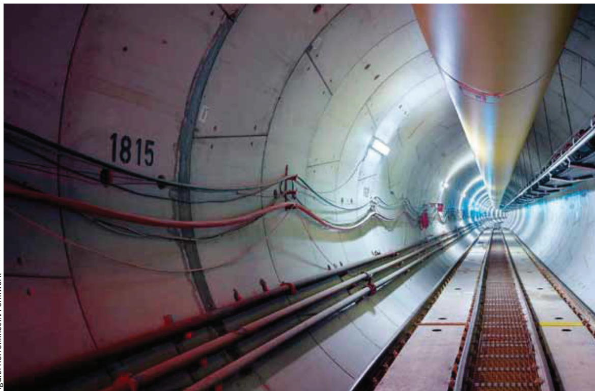
Figure: Herrenknecht Formwork
