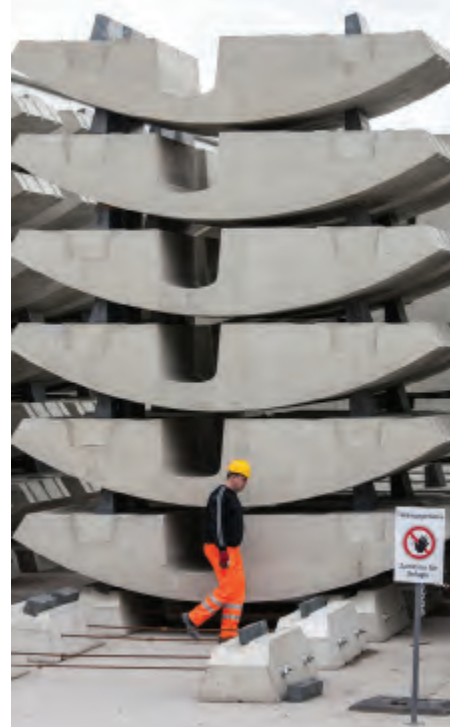
Above: the invert. Top left: segments delivered to the base of the shaft. Top right: segment installation at the TBM
