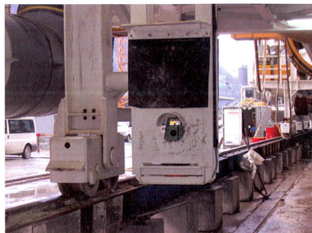
Abb. 2: Totalstation Gotthard-Nord.
