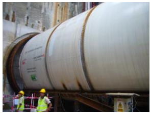
Launching of the TBM in Start Shaft
