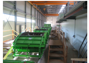
Production line for the segments
