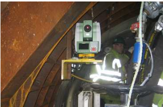
Installed Hardware of Navigation System
